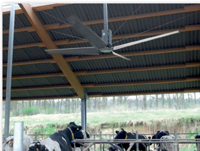
Figure 7: Typical arrangement of ceiling fans (source: Pelzer)
