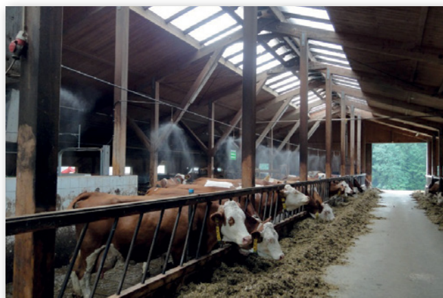
Figure 13: Example of a high-pressure atomisation system (source: Zahner)
